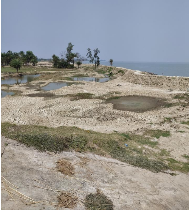
Photo 4.9: Damaged farm lands from saline water ingress after embankment breach in Sagar island
